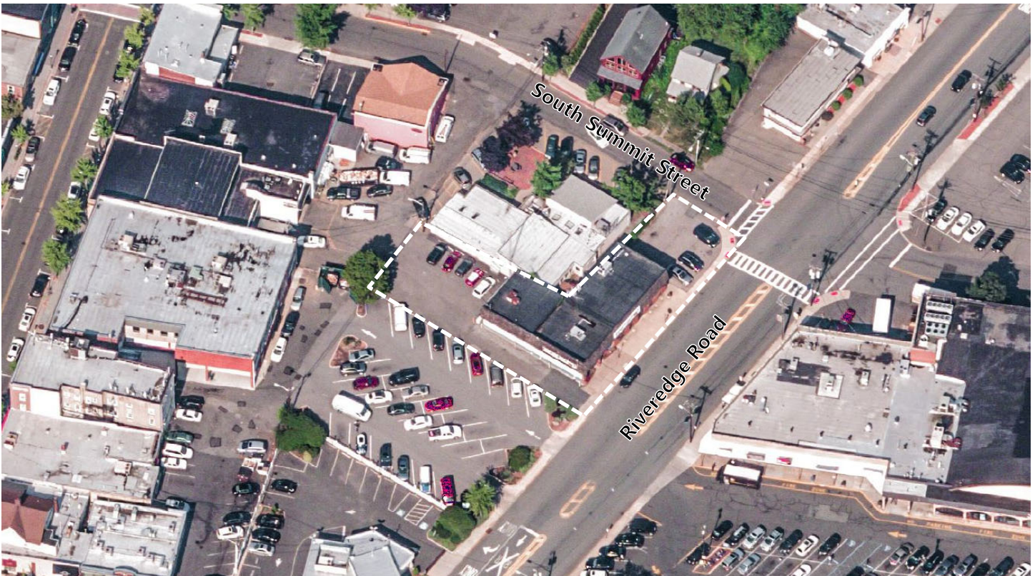
Figure 8: South Summit Street/Riveredge Road Overlay Site, Looking West (Source: Bing Maps. Note: Lot Lines Approximate)
