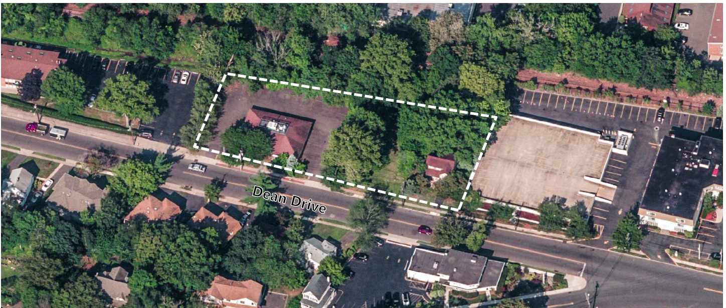
Figure 1: Dean Drive Site, Looking West (source: Bing Maps. Note: Lot Lines Approximate)
